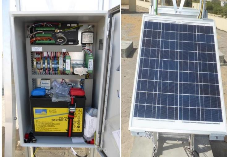
Fig. 6: Control box with data logger, battery and electric equipment
